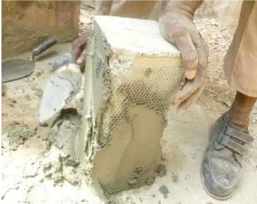
Plate 3. 62: Applyingmortaroncolumn surface
