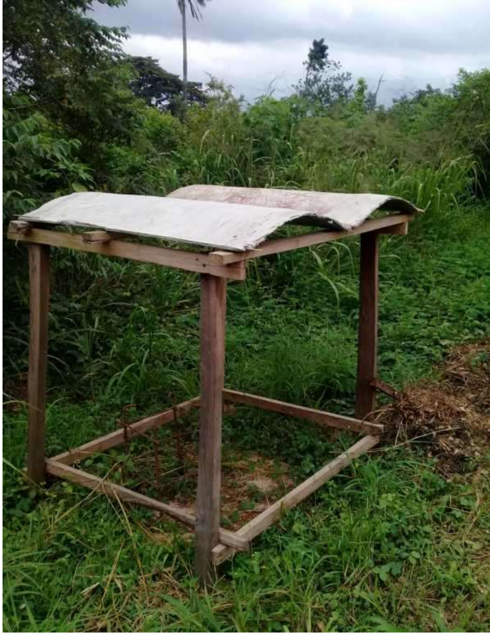
Plate 3.9: Developed ferrocement roof installed in the Faculty of Technology, University of Ibadan.
