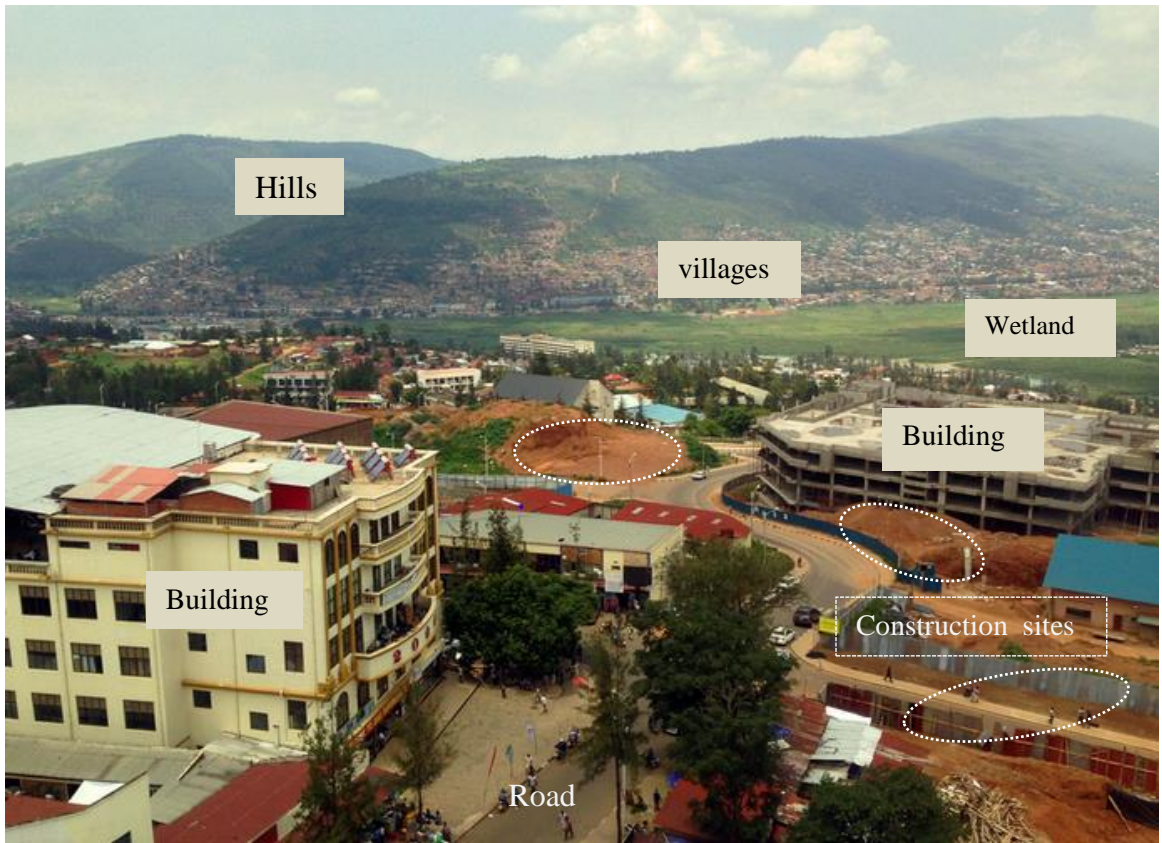
Figure 1.3 Environment condition of Kigali city.
