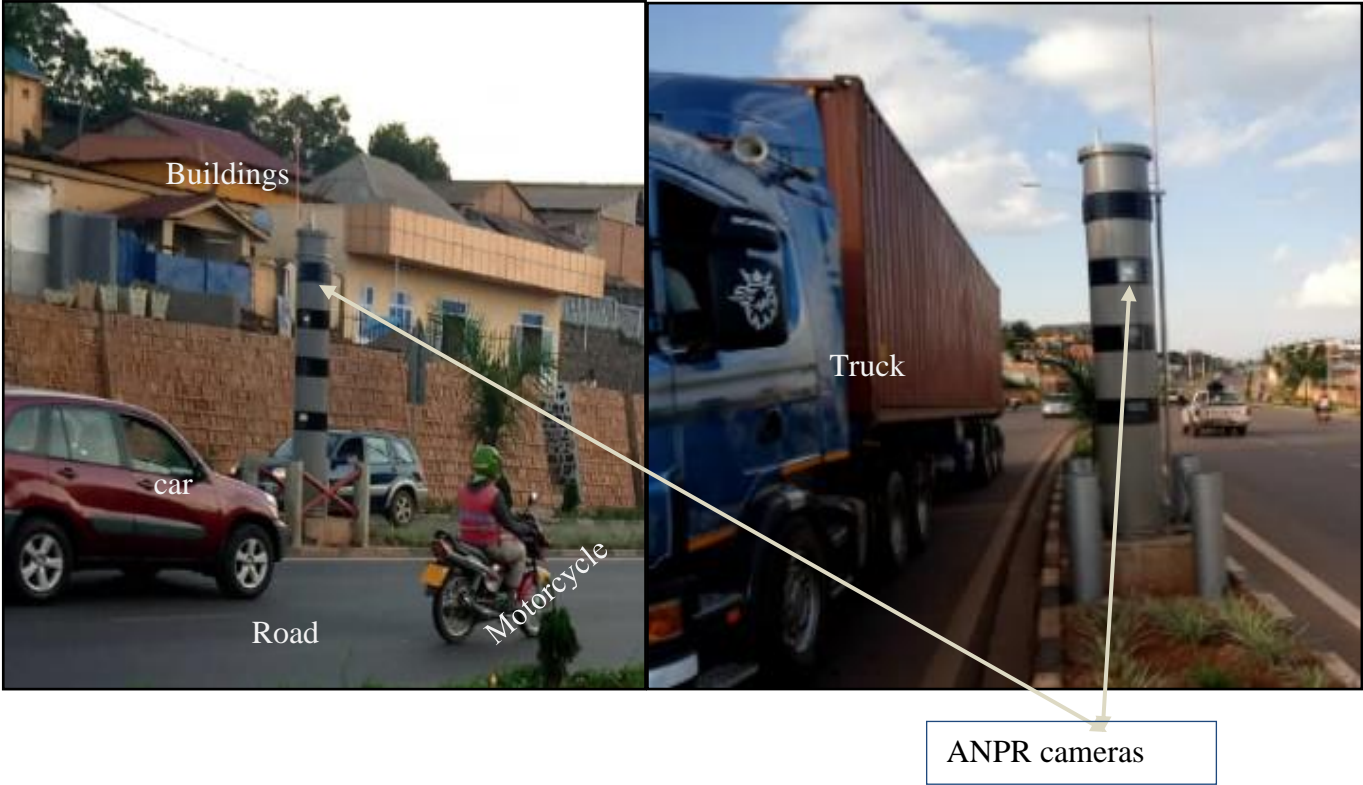
Figure 1.4 The existing ANPR cameras installed in Kigali
