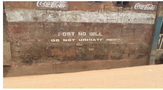
A monophonic public road sign
