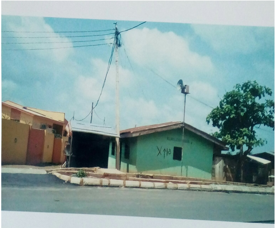
Plate 5: A Mosque showing loudspeakers mounted on its top located in residential area, Sharp Corner, Apata, Ibadan.
