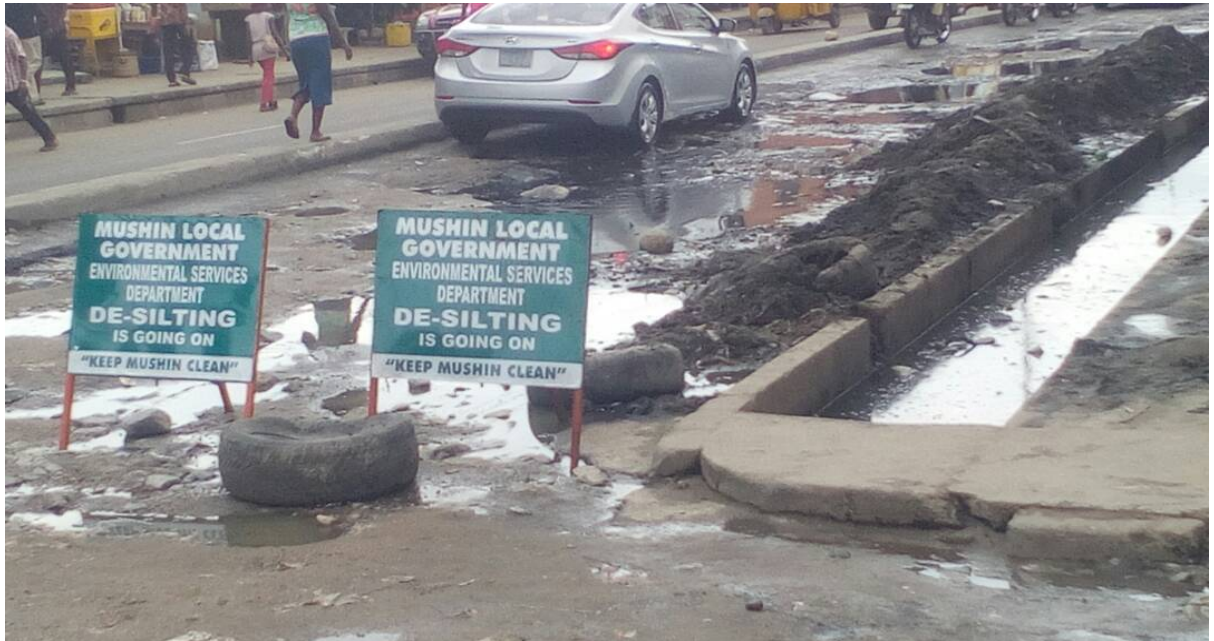
Plate 7: De-silting of drainages by the Mushin Local Government Environmental Unit
